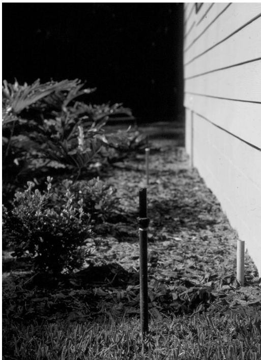
FIGURE A.17.1.8.1(b) Use of Low Volume Sprinklers in Organic Material. [1144:Figure A.4.2.4.1(b)]
