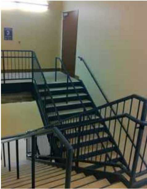
An enclosed stair that constitutes an exit.
