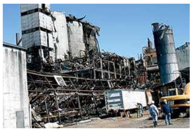
(Courtesy of the U.S. Chemical Safety Board)
