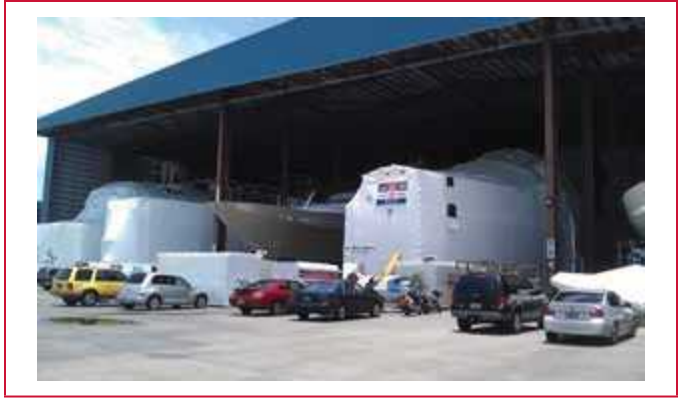
Temporary membrane enclosures surrounding motor yachts. (Courtesy of Global Finishing Solutions)
