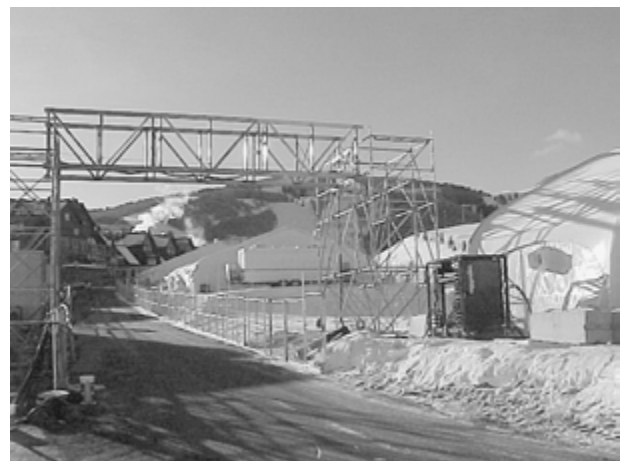
Elevated electrical system.
