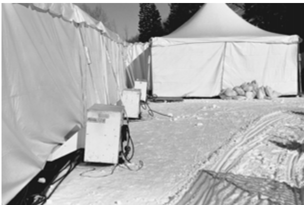
Portable heaters placed outside membrane structure.
