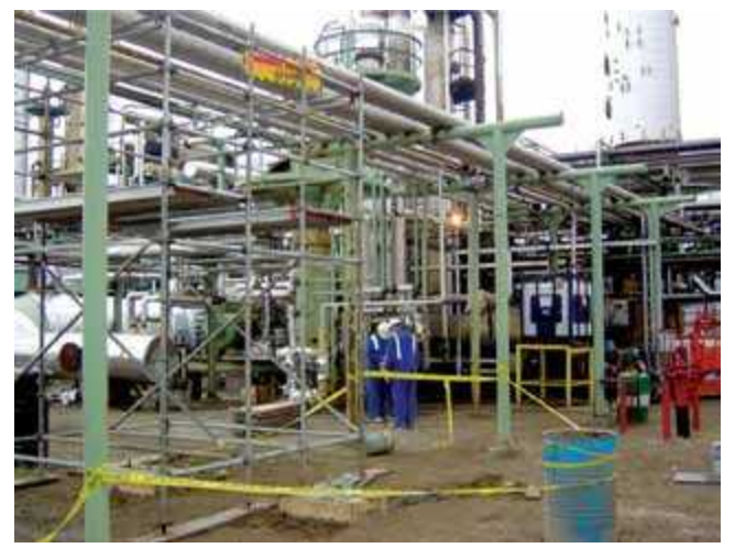
Piping in a process plant undergoing routine maintenance.
