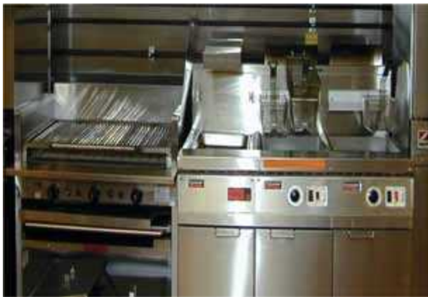
Example of a baffle plate providing separation between a fryer and an adjacent appliance that produces surface flames.
