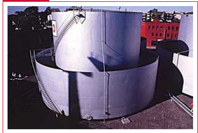
Diked tank to which 66.22.11.2.5(1) applies.
