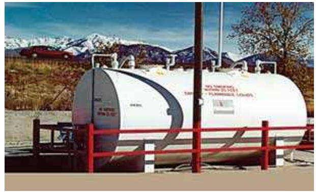
Collision protection for an aboveground storage tank. (Courtesy of Steel Tank Institute)
