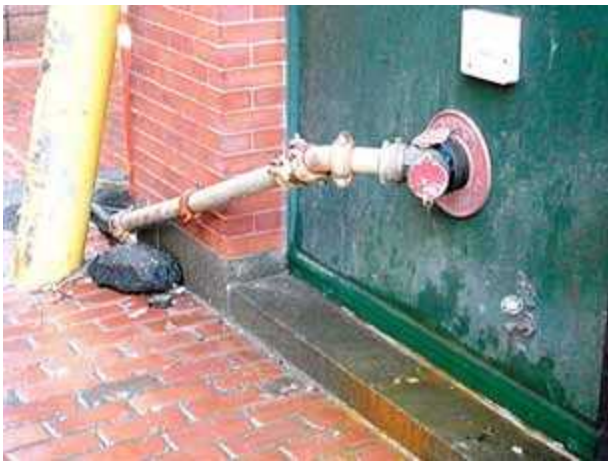
Temporary water supply connection to FDC.
