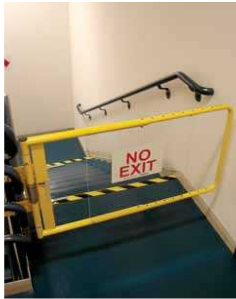
Sign on gate providing interruption of exit stair. (Courtesy of Jake Pauls)
