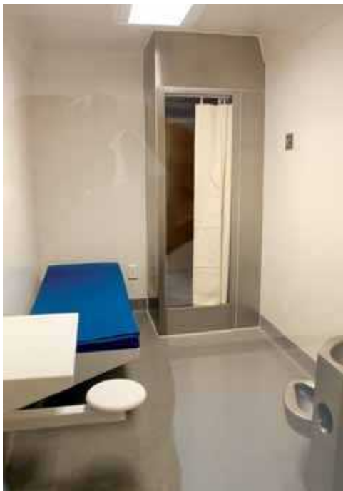
Resident room with interior wall and ceiling finishes that do not pose a fire spread problem.
