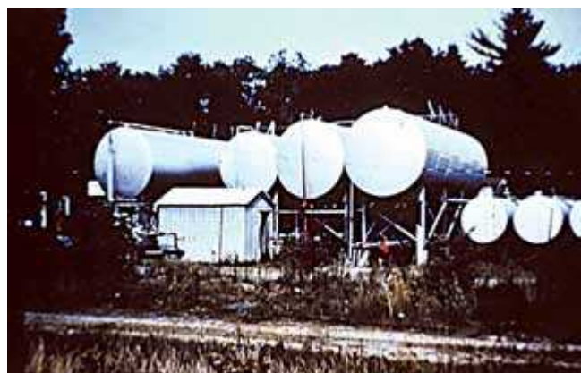
Aboveground tanks on unprotected steel supports (left). Aftermath of a fire where tanks were supported on unprotected steel supports (right).
