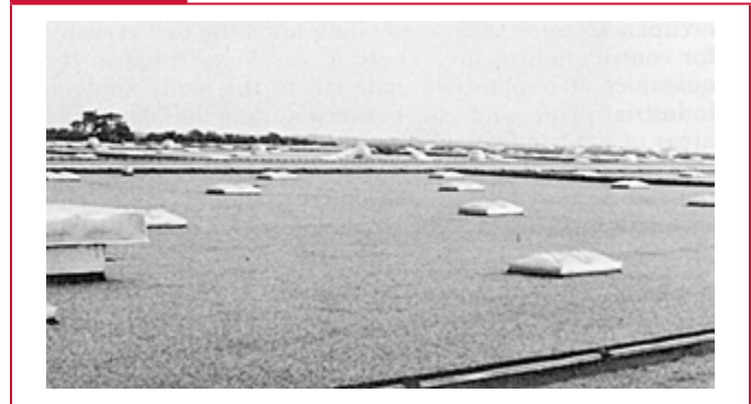
View of roof vents on building.
