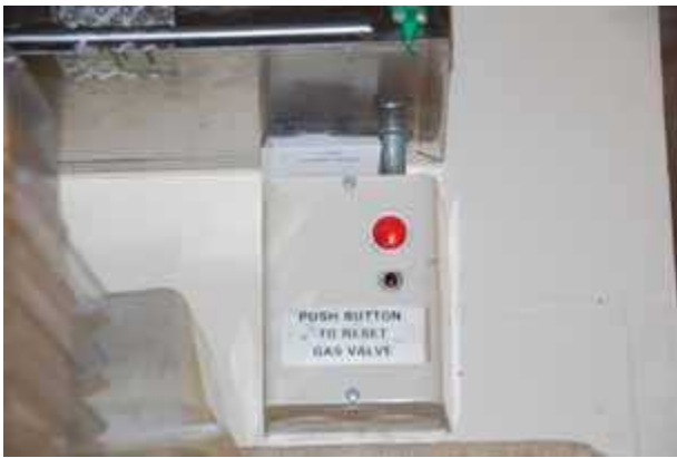
Manual reset for fuel and electric power.
