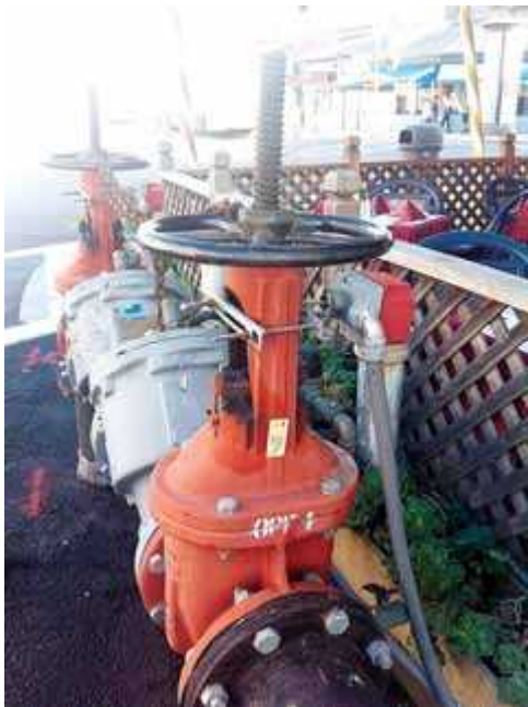
Outside screw and yoke (OS&Y) gate valve.
