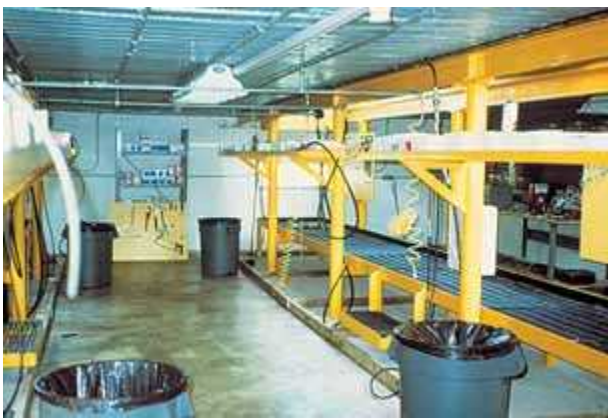
Belowgrade work area of a lube-only facility. (Courtesy of Jiffy-Lube)
