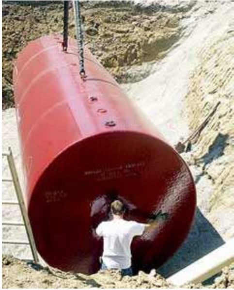
Installation of an underground tank. (Courtesy of Fairfield Ledger)
