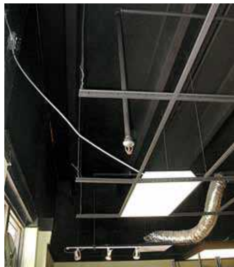
No drop ceiling. (Courtesy of Byron Blake and SimplexGrinnell)
