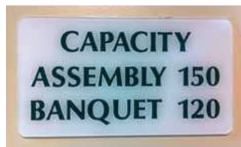
Typical occupant load signage for an assembly occupancy.
