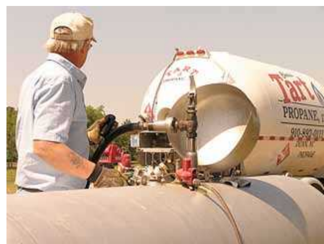
Filling a storage container. (Courtesy of Richard Fredenburg and Tart Propane)
