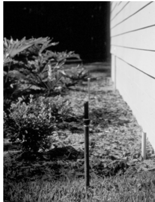
FIGURE A.17.1.8.1(b) Use of Low Volume Sprinklers in Organic Material. [1144:Figure A.4.2.4.1(b)]
