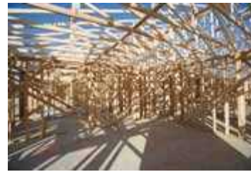
(e) Type V construction
