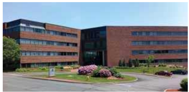
Typical business occupancy building.
