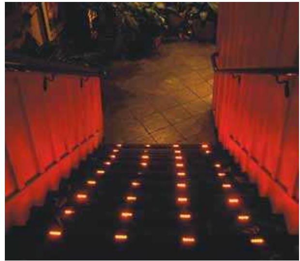
Interior stair illumination via lights at stair treads. (Courtesy of Jake Pauls)
