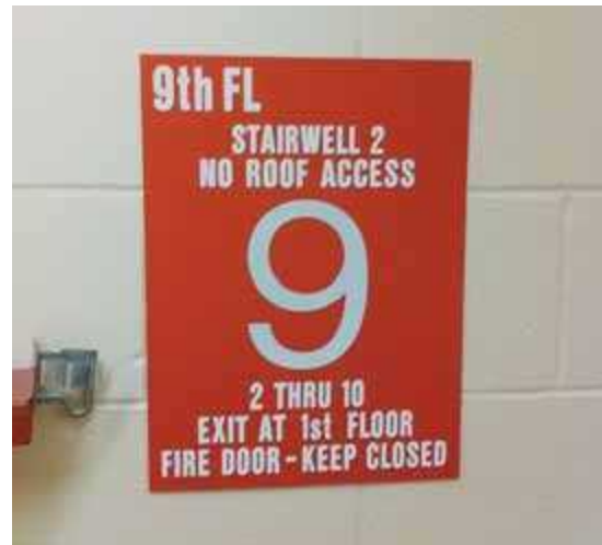
Stairway identification sign with tactile floor level designator.
