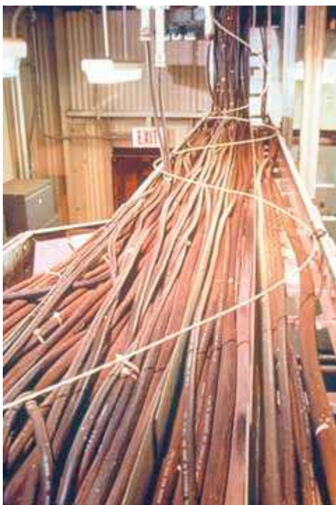
Line-type heat detector installed in a cable tray application. (Source: The Protectowire Co., Inc., Pembroke, MA)
