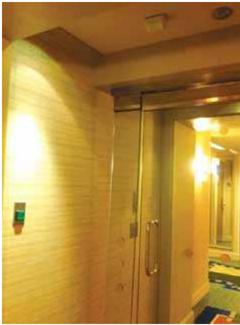
Egress side of sensor-release of electrical locking system door assembly.
