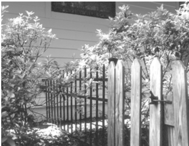
FIGURE A.17.1.8.3(b) Transition Fence Separates Combustible Fence from Structure. (Courtesy of Firewise Communities Program. Photo by G. Johnston.) [1144:Figure A.4.2.4.3(b)]
