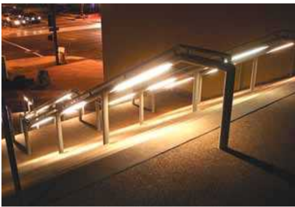
Exterior stair illumination via lights in stair handrail. (Courtesy of Jake Pauls)
