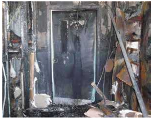
Fire door assembly from fire side.
