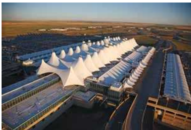
Membrane structure. (Courtesy of Denver International Airport)
