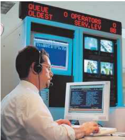
Central Station with Display in Background Indicating Signal Traffic and Availability to Process Incoming Signals. (Source: SimplexGrinnell, Westminster, MA)
