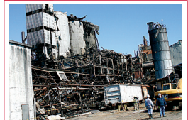
(Courtesy of the U.S. Chemical Safety Board)
