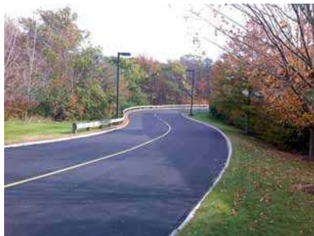
Fire department access road.
