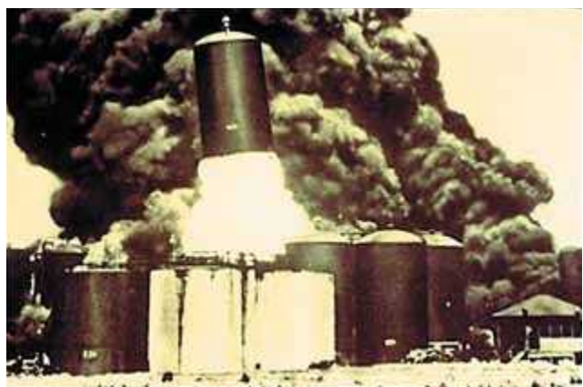
Catastrophic failure and rocketing of a tank due to inadequate emergency relief venting.
