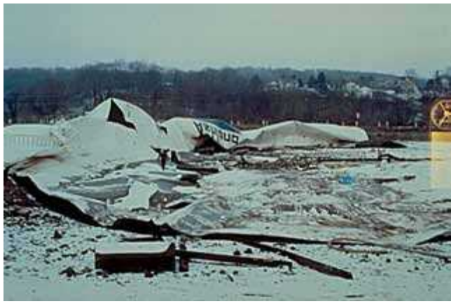
Destroyed oil storage tank, Floreffe, Pennsylvania, January 2, 1988.
