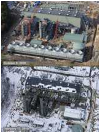
Kleen Energy plant before and after explosion. (Source: U.S. Chemical Safety Board)
