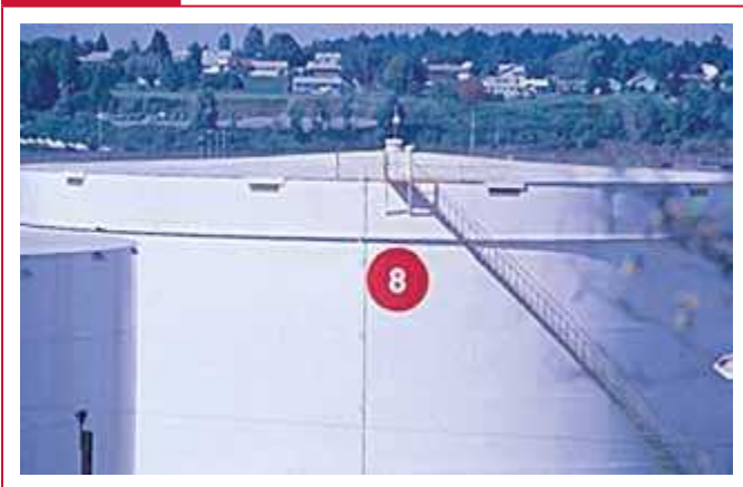
Closed-top floating roof tank.
