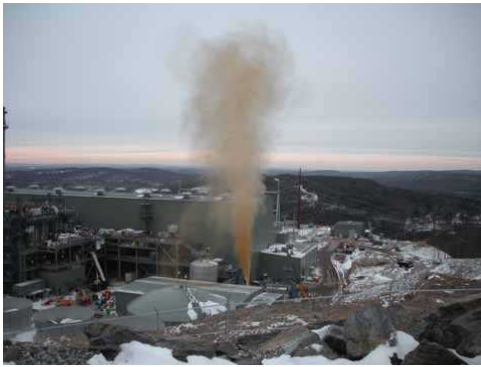
Gas blow. (Source: U.S. Chemical Safety Board)
