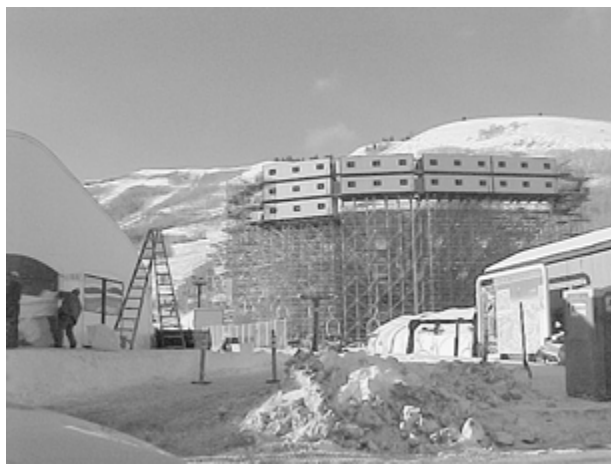
Temporary grandstand with enclosed spaces above.
