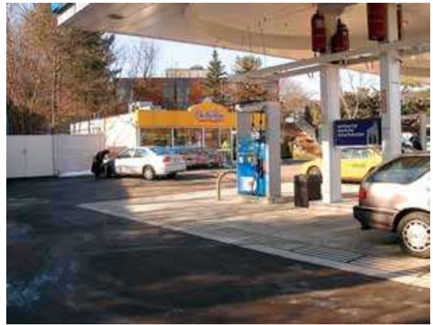
Typical service station and convenience store.
