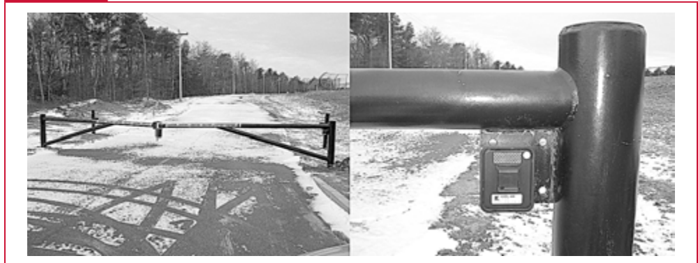
Example of gate access and access box.
