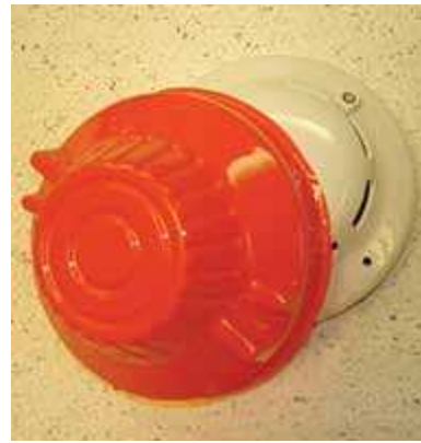
Smoke detector with protective plastic cover. (Courtesy of Hochiki America Corp., Buena Park, CA)
