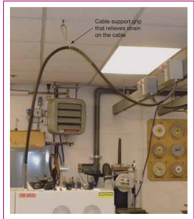
EXHIBIT 368.3 An example of a cable or cord branch from a busway installed according to 368.56(B).
