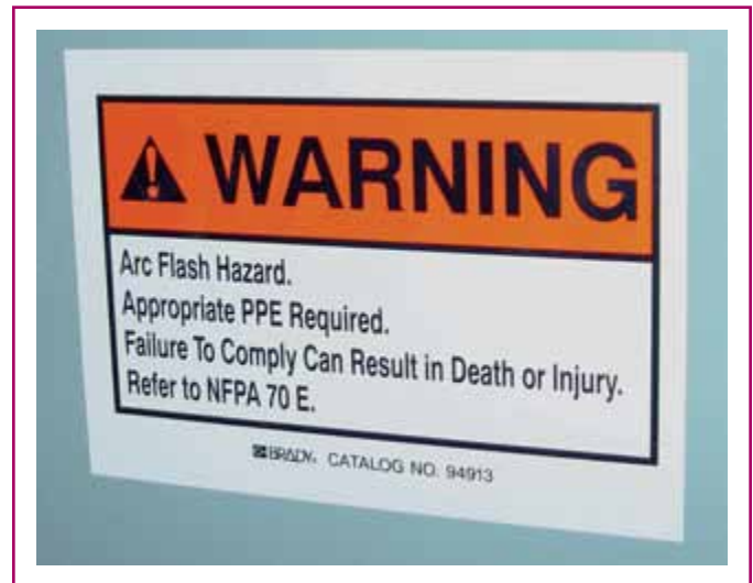
EXHIBIT 110.8 One example of an arc-flash warning sign. (Courtesy of the International Association of Electrical Inspectors)
