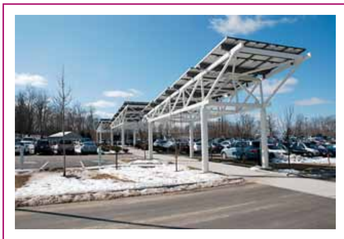
EXHIBIT 690.2 A PV array support structure that allows for continued use of the walkway. (Courtesy of Solar Design Associates, LLC)
