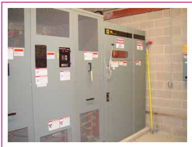
EXHIBIT 110.29 Enclosures of equipment operations at over 1000 volts required to have the warning label specified in 110.31(B)(1) . (Courtesy of the International Association of Electrical Inspectors)
