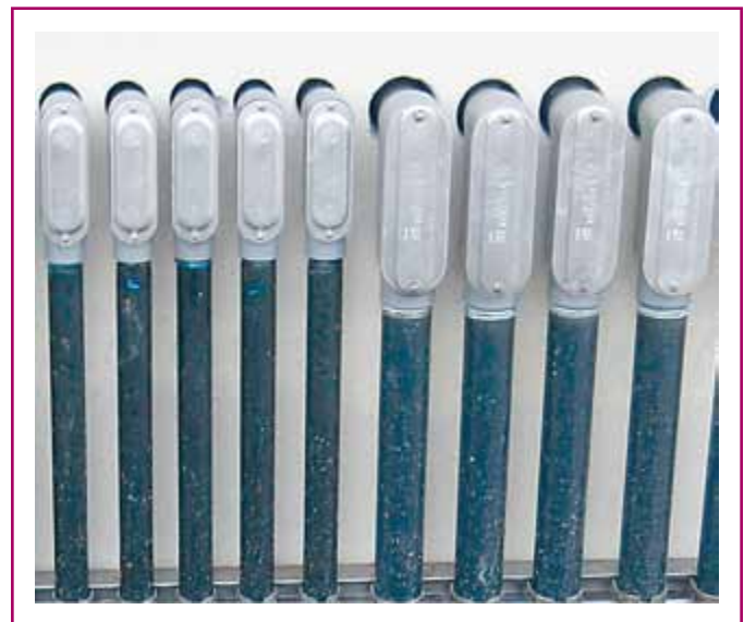
EXHIBIT 100.9 Typical conduit bodies. (Courtesy of the National Electrical Contractors Association)
