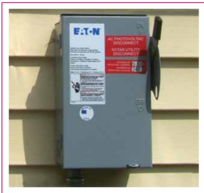
EXHIBIT 690.10 PV system disconnect.
