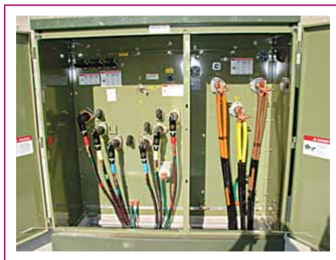
EXHIBIT 490.3 Open view of a tamperproof pad-mounted transformer for loop-feed application with load-break elbow connectors. (Courtesy of Schneider Electric)
