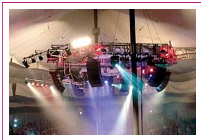
EXHIBIT 520.6 A suspended border light assembly over a stage.
