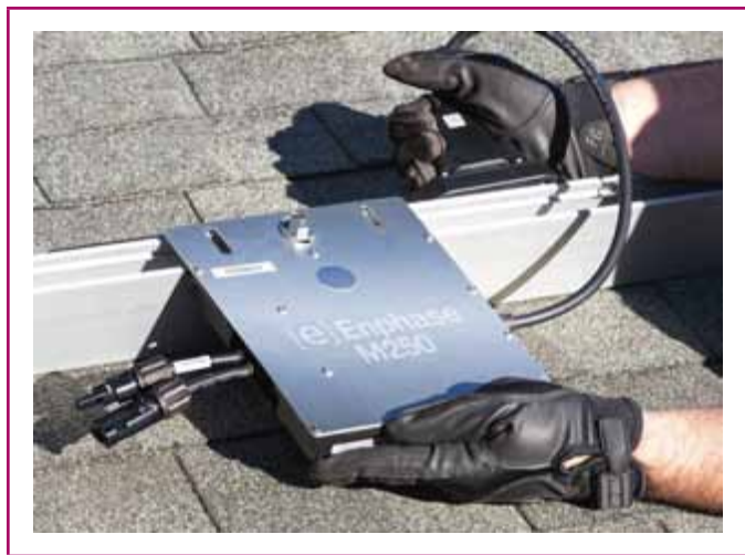
EXHIBIT 690.4 A microinverter with connectors meeting the requirements of 690.33. (Courtesy of Enphase Energy)
