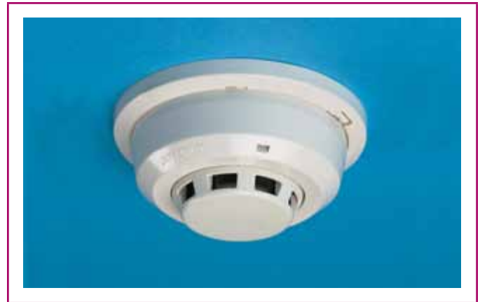
EXHIBIT 760.2 Typical spot-type smoke detector.
