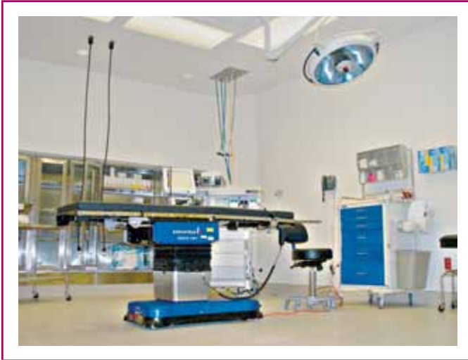
EXHIBIT 517.1 An operating room where patients are connected to line-operated electromedical devices while undergoing invasive procedures. (Courtesy of the International Association of Electrical Inspectors)
