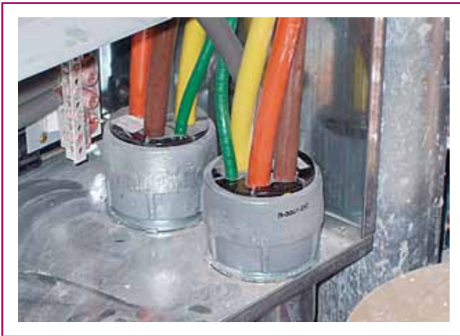
EXHIBIT 300.16 A support bushing, located at the top of a vertical conduit at a cabinet or pull box, used to prevent the weight of the conductors from damaging insulation or placing strain on termination points.
