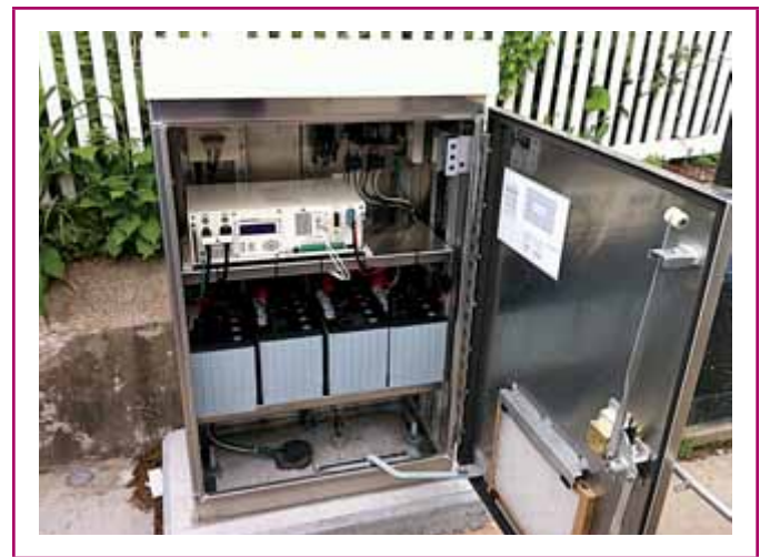
EXHIBIT 690.5 Stand-alone system components. (Courtesy of Solar Design Associates, LLC)
