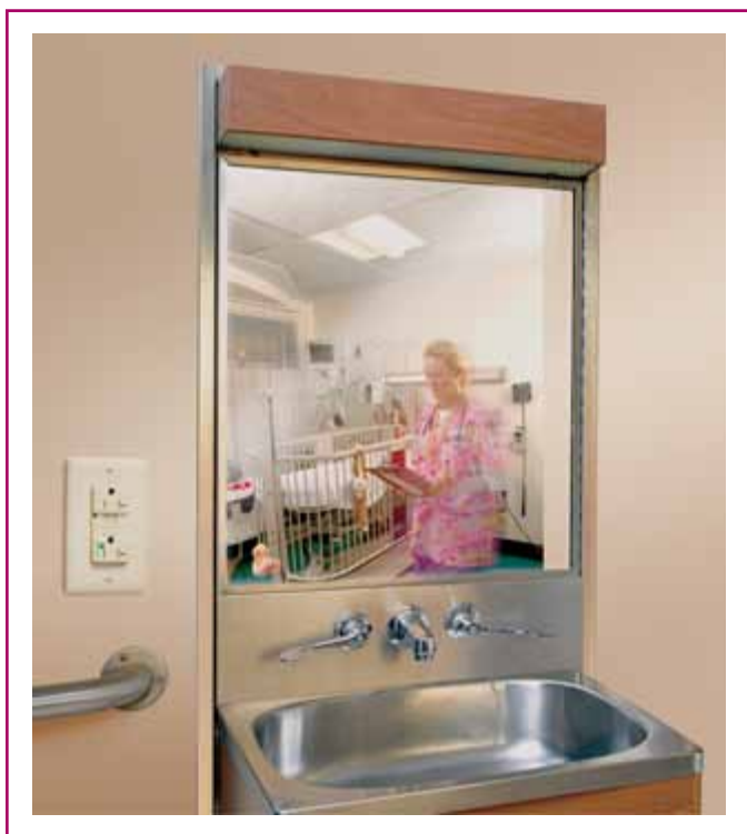
EXHIBIT 517.3 Hospital-grade, tamper-resistant GFCI in a hospital environment. (Courtesy of Legrand®)
