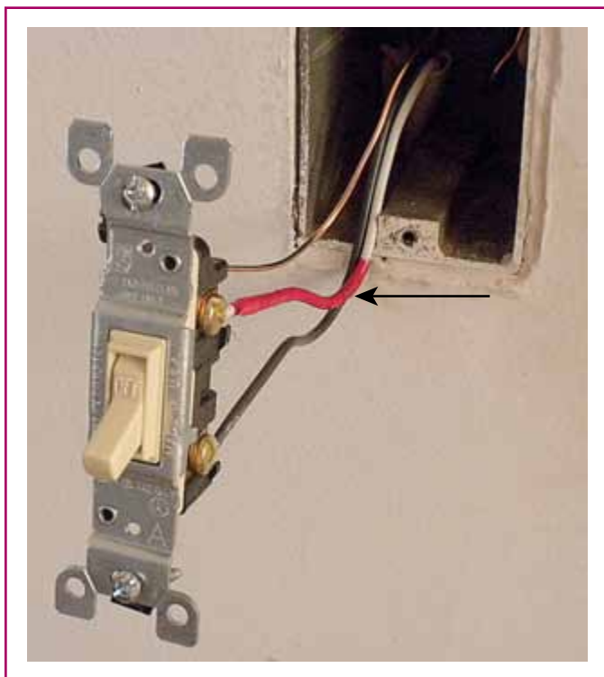
EXHIBIT 200.5 The re-identified conductor at a switch location, limited to use only as the ungrounded conductor that supplies the switch.
