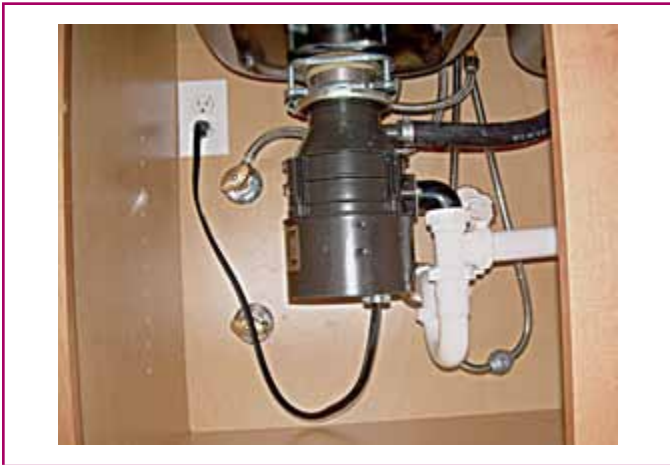
EXHIBIT 422.2 A cord-and-plug-connected kitchen waste disposer. (Courtesy of the National Electrical Contractors Association)
