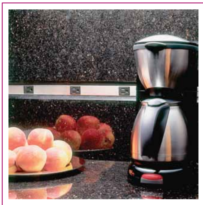
EXHIBIT 100.13 A multioutlet assembly installed to serve countertop appliances. (Courtesy of Legrand/Wiremold®)
