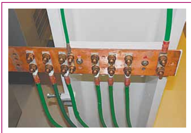
EXHIBIT 250.17 Listed connectors used to connect the common grounding electrode conductor and individual taps to a centrally located copper busbar with a minimum dimension of ¼ inch thick by 2 inches wide.
