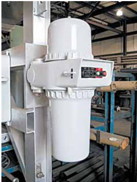
EXHIBIT 501.14 An explosionproof enclosure for a motor control starter and circuit breaker. (Courtesy of Appleton®, Emerson Electric Co.)
