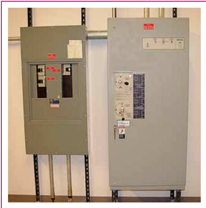
EXHIBIT 700.1 An emergency system transfer switch. (Courtesy of the International Association of Electrical Inspectors)
