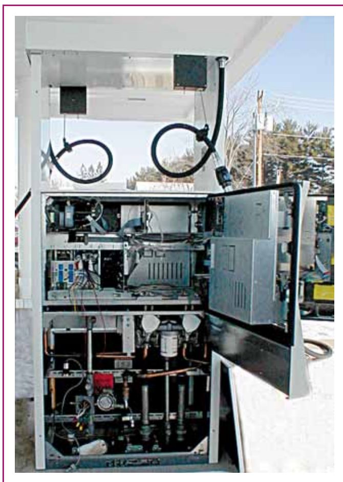
EXHIBIT 514.7 An example of the complexity of the interior of electronic dispensing units.
