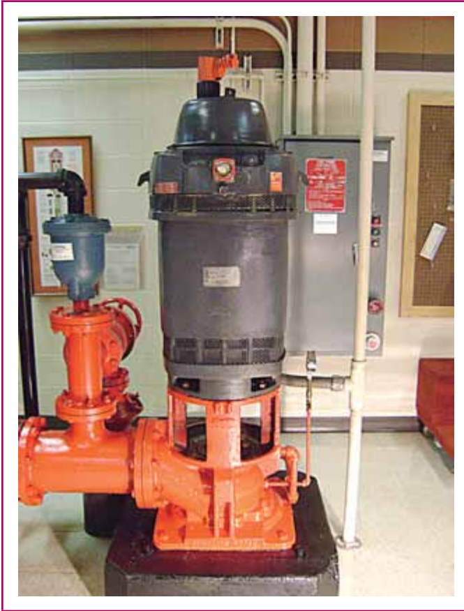
EXHIBIT 695.1 An electric motor specifically listed for fire pump service. (Courtesy of Liberty Mutual Insurance)
