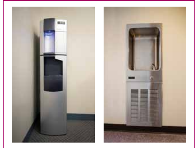
EXHIBIT 422.1 Two types of electrically powered water coolers required to have GFCI protection.
