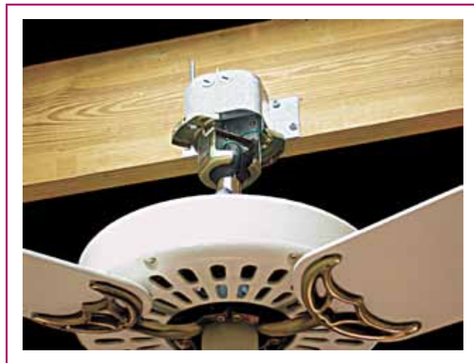
EXHIBIT 422.3 Supporting a ceiling-suspended (paddle) fan (35 pounds or less) with a box identified for such use. (Courtesy of Hubbell Incorporated)
