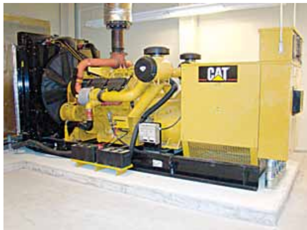
EXHIBIT 445.1 A diesel engine-driven generator that may be used in an emergency system, legally required standby system, optional standby system, or critical operations standby system.
