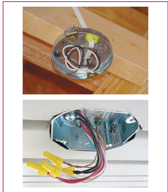
EXHIBIT 314.9 Two methods of supporting a ceiling fan from a listed outlet box. (Top) A listed outlet box used as the sole support of a ceiling-suspended (paddle) fan. Note the two clamps on the perimeter of the box that will support a fixture. (Courtesy of the International Association of Electrical Inspectors). (Bottom) A box listed for supporting a ceiling-suspended (paddle) fan (35 pounds or less) (Courtesy of Hubbell Incorporated)
