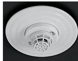
Fixed-Temperature (Nonrestorable) Heat Detector. (Source: Kidde-Fenwal, Ashland, MA)
