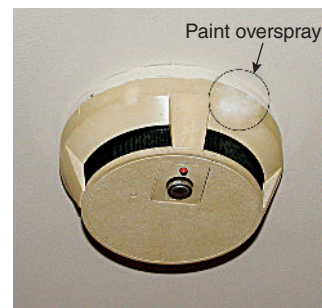
Initiating Device Showing Signs of Paint Overspray, and the Device Is in Alarm. (Courtesy of Jeffrey Moore, P.E., JENSEN HUGHES)
