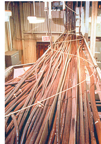
Line-Type Heat Detector Installed in a Cable Tray Application. (Source: The Protectowire Co., Inc., Pembroke, MA)
