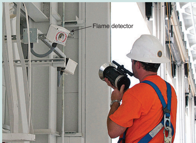
Testing the Response of a Flame Detector. (Courtesy of Jeffrey Moore, P.E., JENSEN HUGHES)
