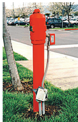
Initiating Device Showing Signs of Paint Overspray, and the Device Is in Alarm. (Courtesy of Jeffrey Moore, P.E., JENSEN HUGHES)
