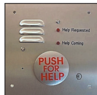
Area of Rescue Assistance Station. (Courtesy of Housing Devices, Inc., Medford, MA)
