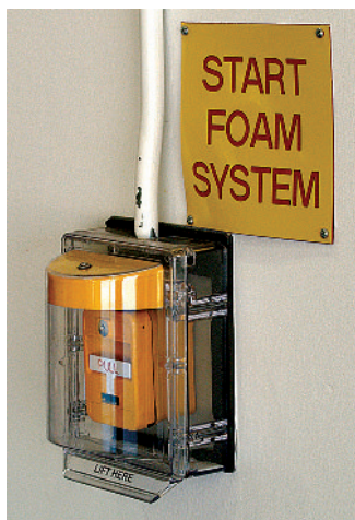
Foam Fire Suppression System Manual Activation Switch. (Courtesy of Jeffrey Moore, P.E., JENSEN HUGHES)
