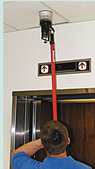
Functional Testing of Smoke Detector. (Courtesy of Jeffrey Moore, P.E., JENSEN HUGHES)
