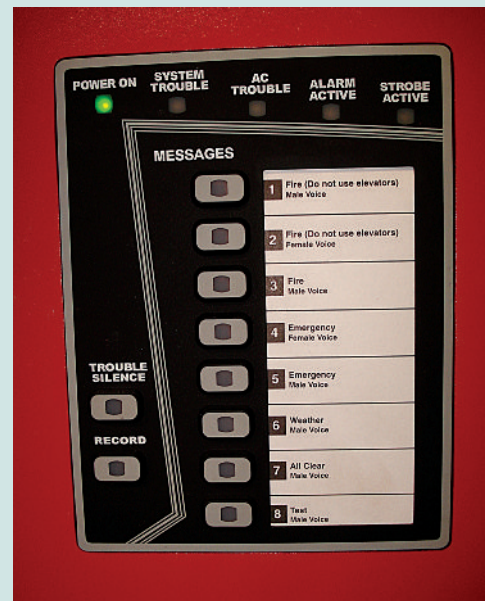
Local Operating Console (LOC) with Preprogrammed Voice Messages. (Courtesy of Jeffrey Moore, P.E., JENSEN HUGHES)
