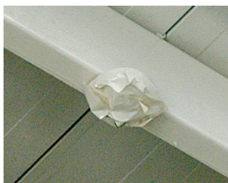
Heat Detector Covered with Tape. (Courtesy of Jeffrey Moore, P.E., JENSEN HUGHES)
