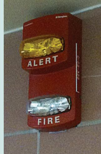
Combination Fire/Alert Visual Notification Appliance.
