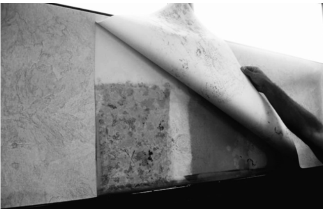
Fig. 4 Impermeable Vinyl Wall Covering on Exterior Wall
