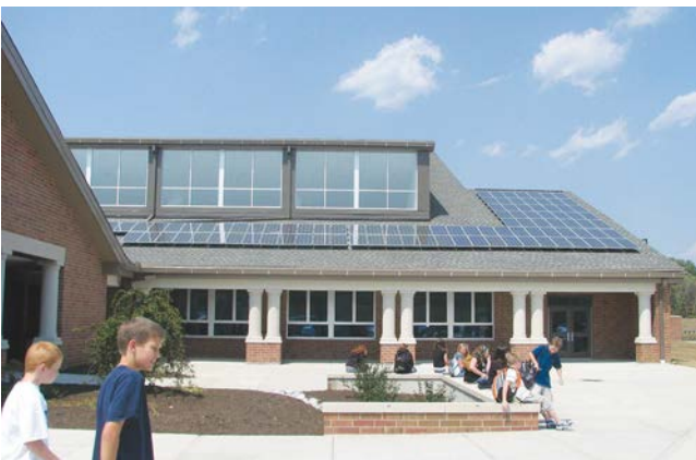
Fig. 10 Example of PV Installation at Twenhofel Middle School, Independence, KY: 22 kW (Seibert 2010)
