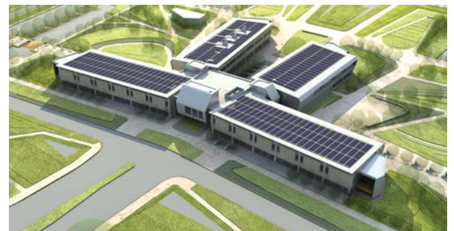
Fig. 9 Example of PV Installation at Ohlone College, Newark Center, Newark, CA: 450 kW, 3530 m 2 (Esberg 2010)
