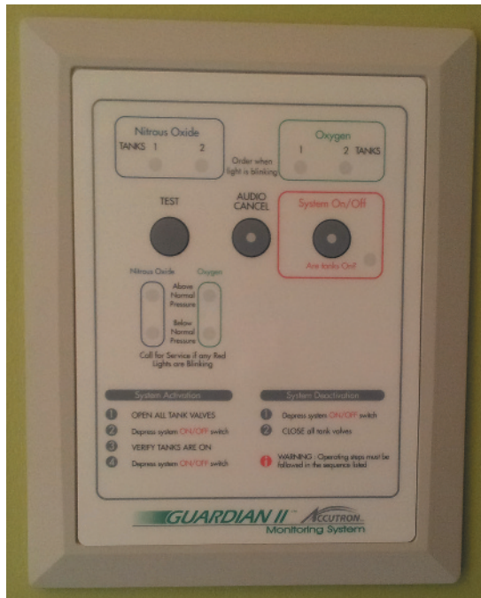
Warning System Alarm Panels for Oxygen and Nitrous Oxide Systems. (Courtesy of William G. Frank Medical Gas Testing & Consulting, LLC)
