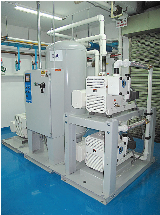
Triplex Vacuum Pump Setup for Piped Medical Vacuum System, Including Control Panel. (Courtesy of BeaconMedaes)
