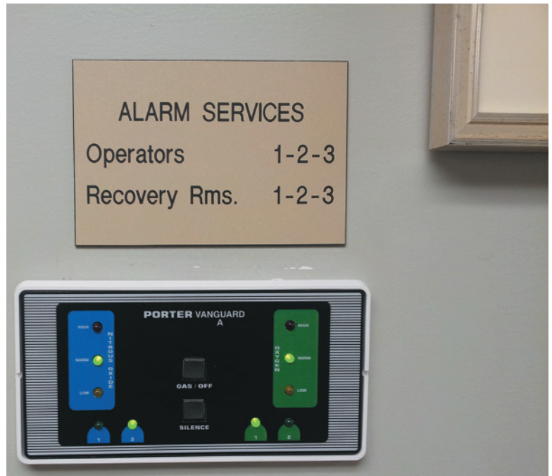
Warning System Alarm Panels for Oxygen and Nitrous Oxide Systems. (Courtesy of William G. Frank Medical Gas Testing & Consulting, LLC)
